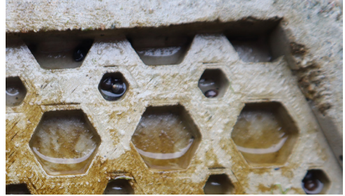
Figure 2. Piling habitat a day after deployment. Already showing the water and sediment retention capability.
